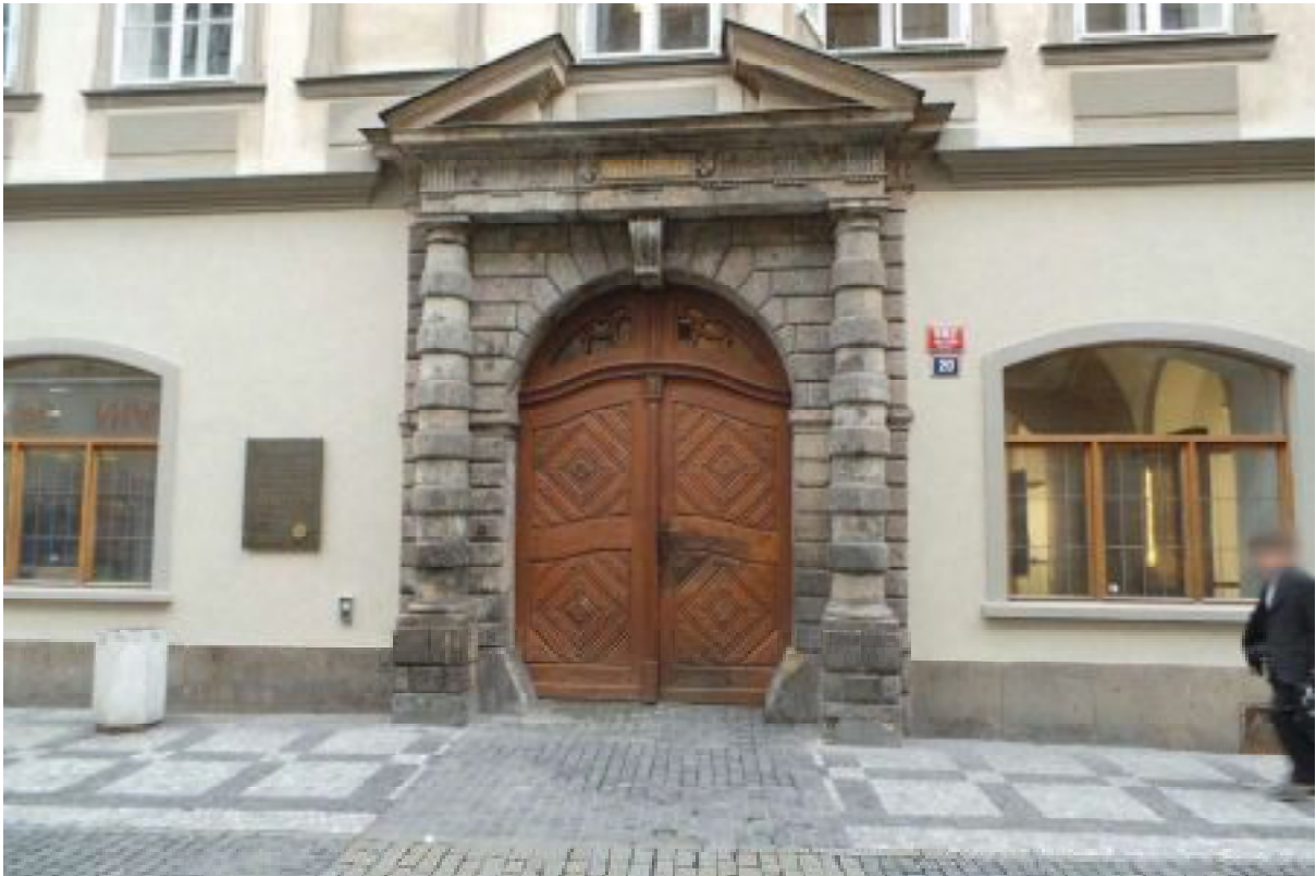
The entrance from the Celetná 20 Street.
